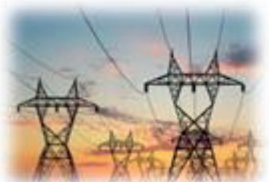
Line 1 Network power
